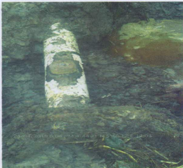
Pic 3.Repair work
