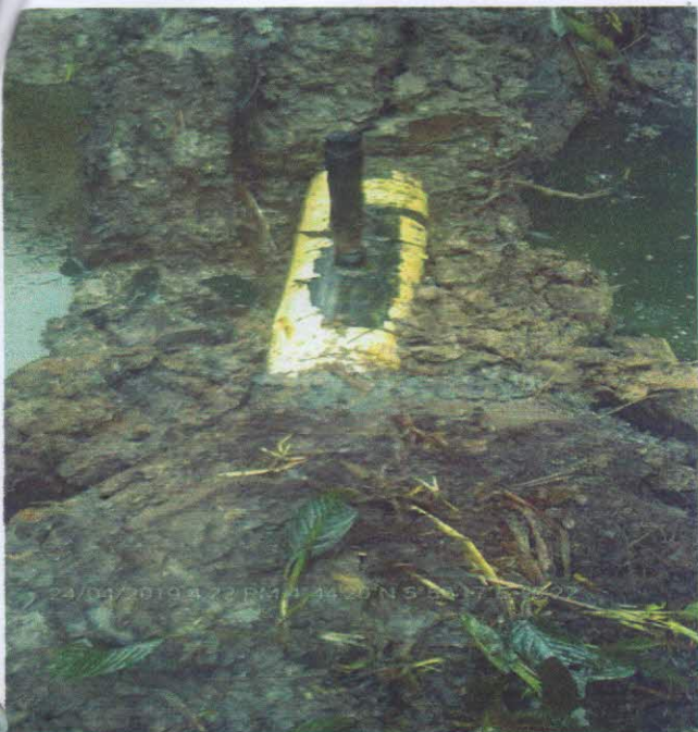
PIC 1. On Excavation
